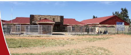
Accommodation Units at Itsoseng Handicraft Centre, constructed at the cost of R34.9m in Ditsobotla Municipality
